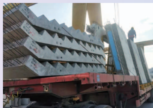
Prefabricated Stair Slabs
