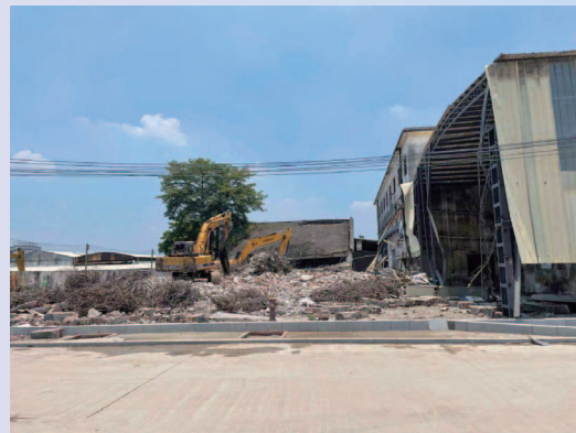
Demolition of Inefficient Industrial Plants
