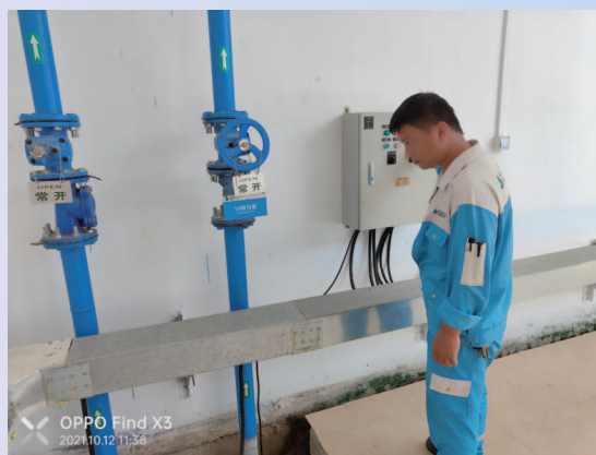
Checking sewage pumps
