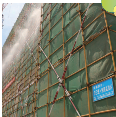
Scaffold Dedusting Spray
