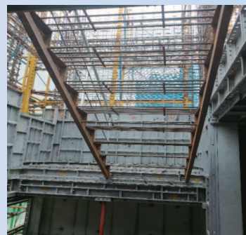
Temporary Ladder Made from Reinforced Steel Remnants
