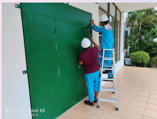
Boarding up doors and windows
